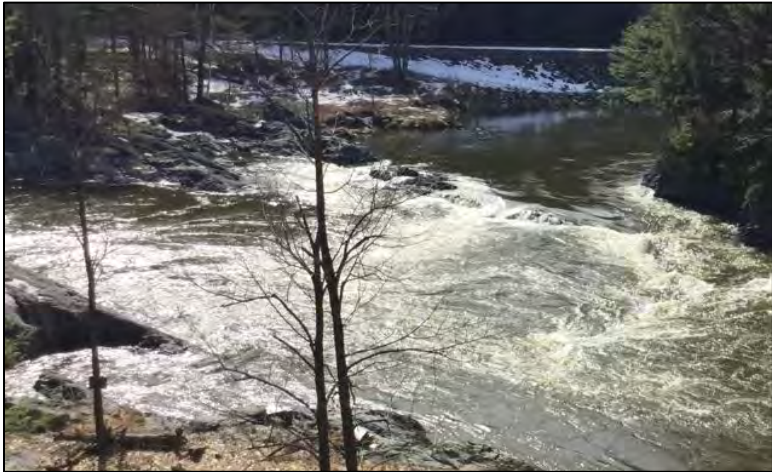
PHOTO 14 RAPIDS DOWNSTREAM OF EAST BARNET DAM (Courtesy of Frank Chaloux)
