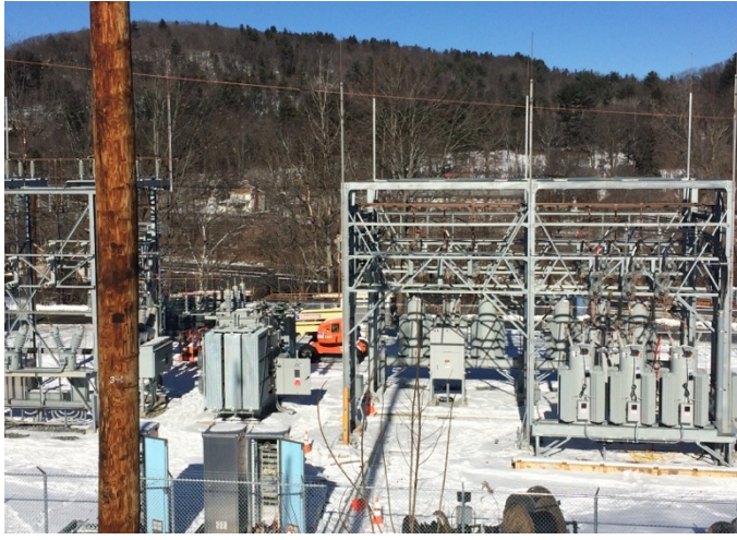
Figure C-4. White River Junction Substation During Construction
