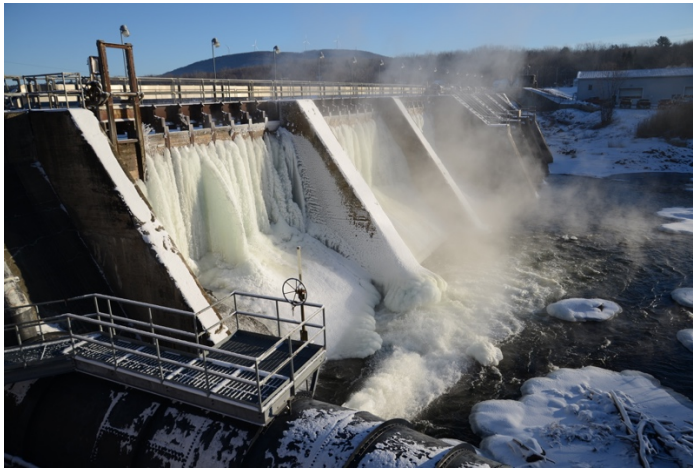
Figure 5-3. Clarks Falls Hydro, Milton
