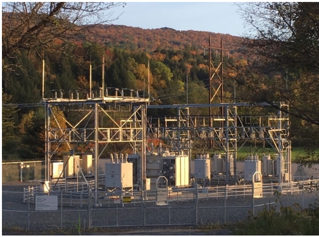
Figure C-3. Waterbury Substation: Relocated and Replaced
