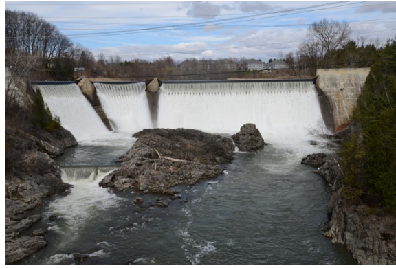
Figure 5-4. Essex #19 Hydro Station
