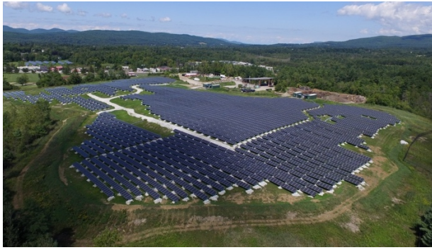
Figure 5-10. Stafford Hill Solar Facility
