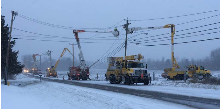
Figure 6-6. Line Crew Restoring a Storm-Related Outage
