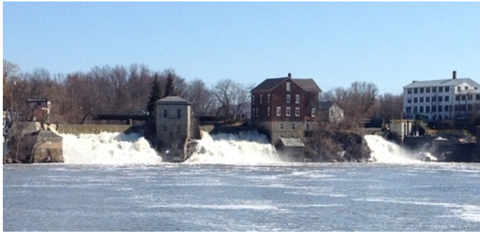
Figure 5-8. Vergennes Hydro Facility
