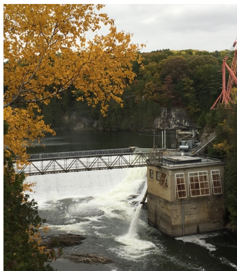
Figure 5-6. Gorge #18 Hydro Facility
